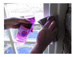
Clean your window frame surfaces, onto which you will be attaching the panel using methylated spirits or a similar degreaser.
